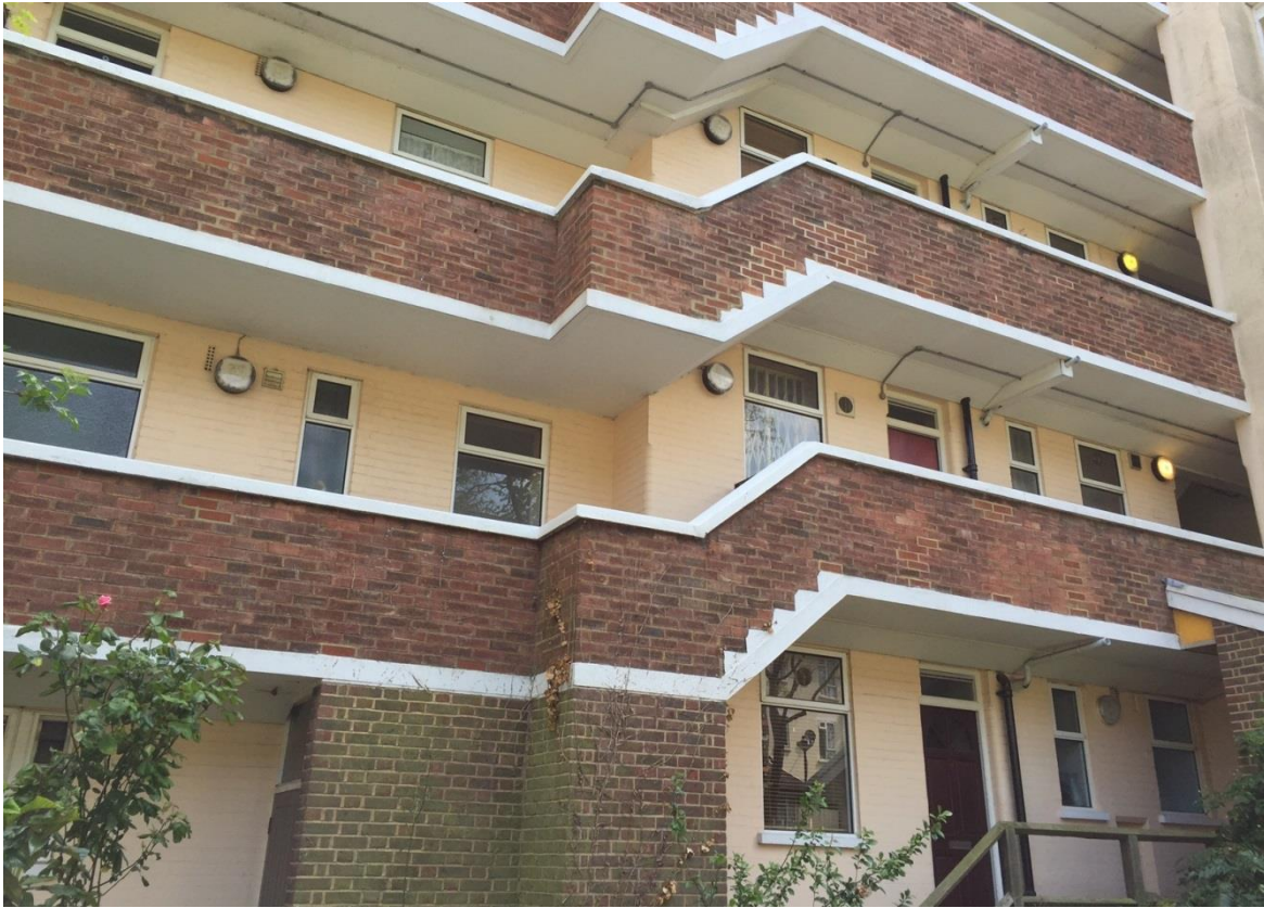
Image 4: North (courtyard) elevation of Mary McArthur House.
