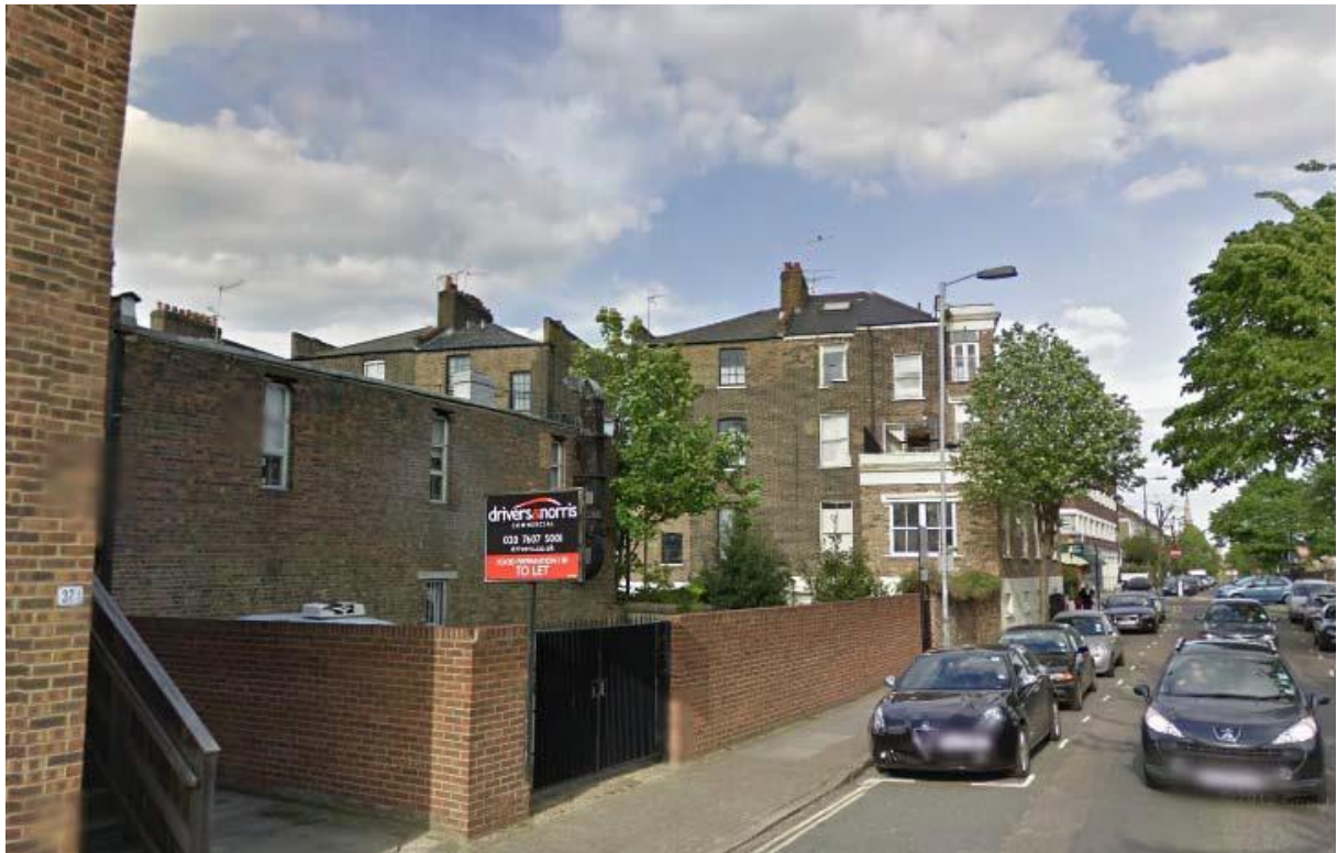
Image 4: view looking to the front of 37 Mildmay Grove North
