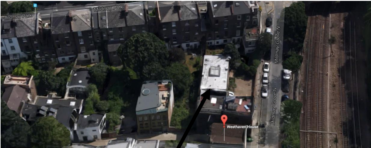
Image 2: Aerial photograph showing the front of 37C Mildmay Grove.
